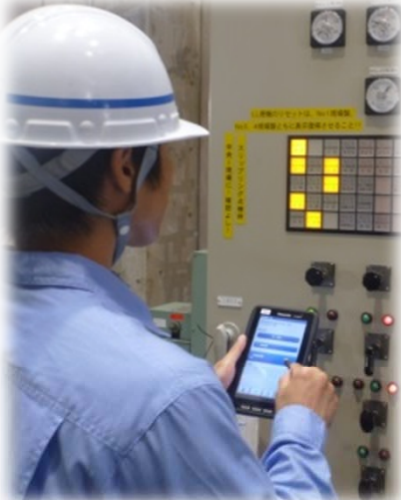
Inspection at site
